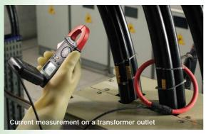
Using a F07 clamp with an Ampflex is an excellent way to combine safety and accessibility on large diameters.
